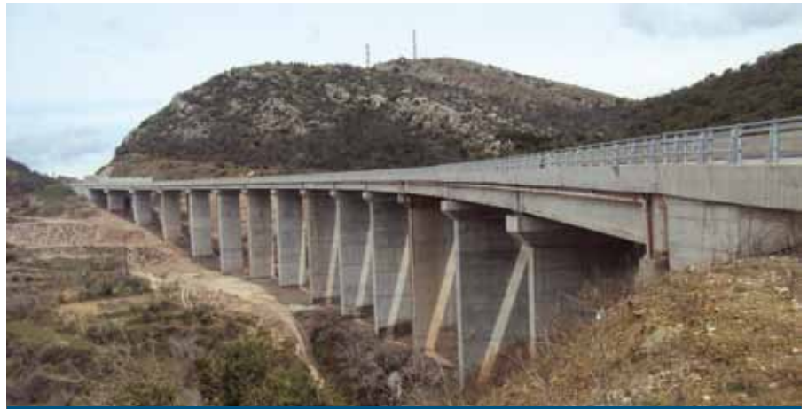
Rehabilitation Works in the National Highway Tripoli-Kalamata, Greece
