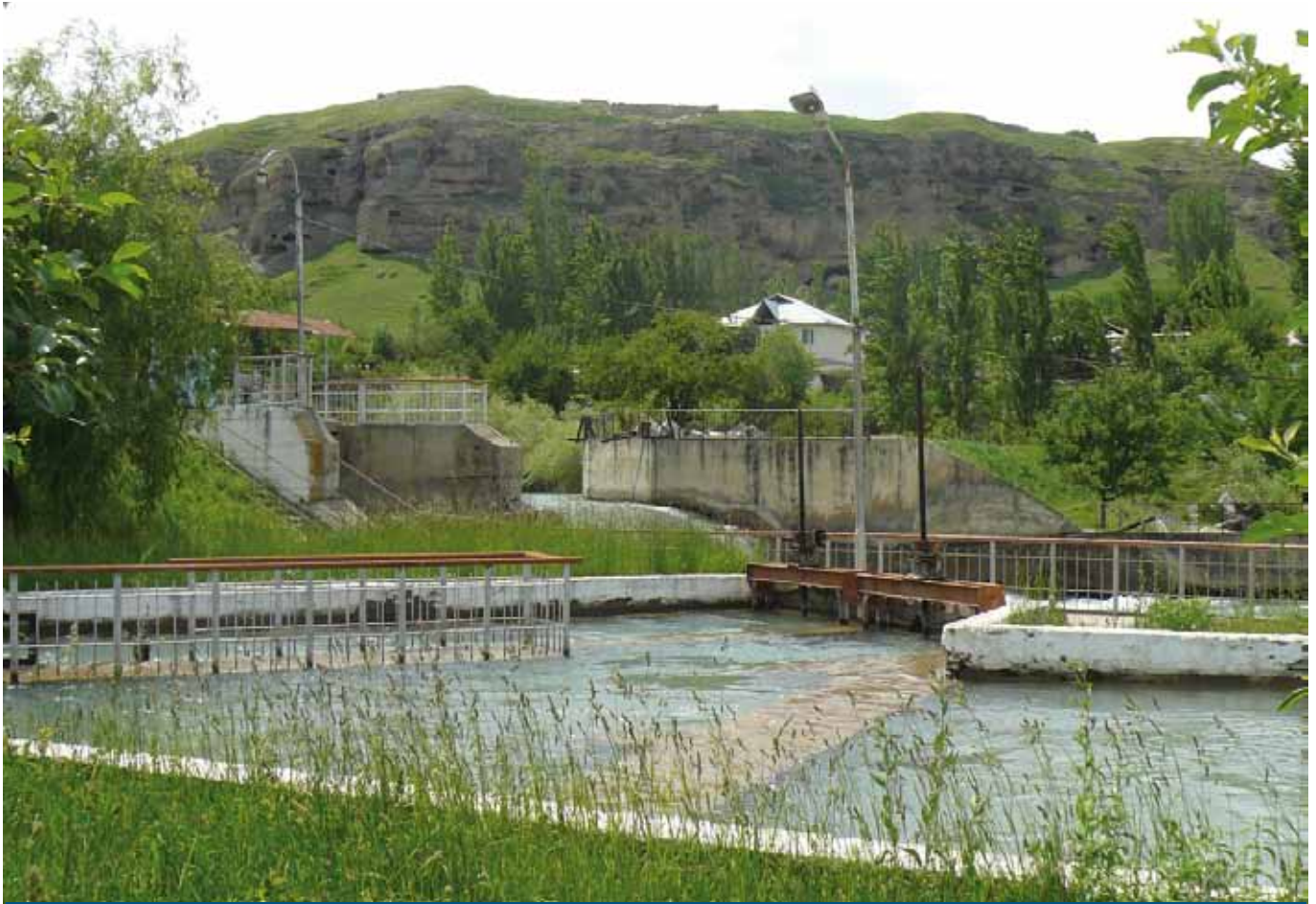
Improvement of the Water Supply and Sanitation Networks in the cities of Osh, Jalal-Abad and Bazar-Korgon, Kyrgyzstan
