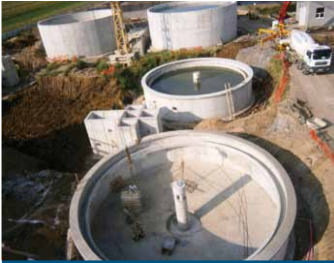
Turnkey project for the Wastewater Treatment Plant in Agnita and Dumbraveni, Romania
