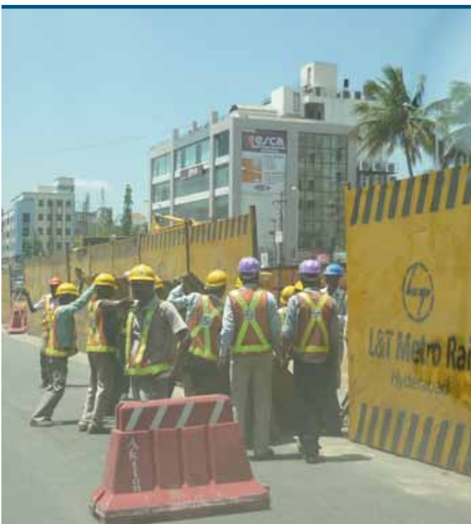
Safety Audit for the Hyderabad Metro, India
