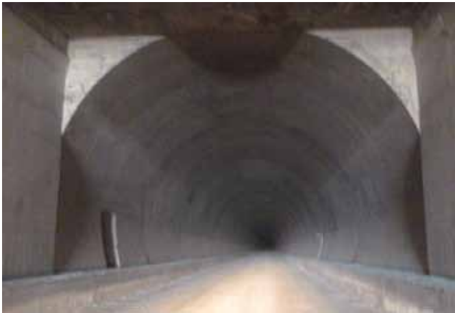
▲ TUNNEL OF AIGIO, E.S.P.EL PROJECT
