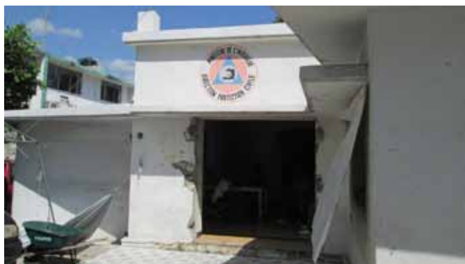
▲ STUDY AND CONSTRUCTION SUPERVISION OF THE MULTIFUNCTIONAL CENTRE FOR THE CIVIL PROTECTION DEPARTMENT IN PORT-AU-PRINCE IN HAITI
