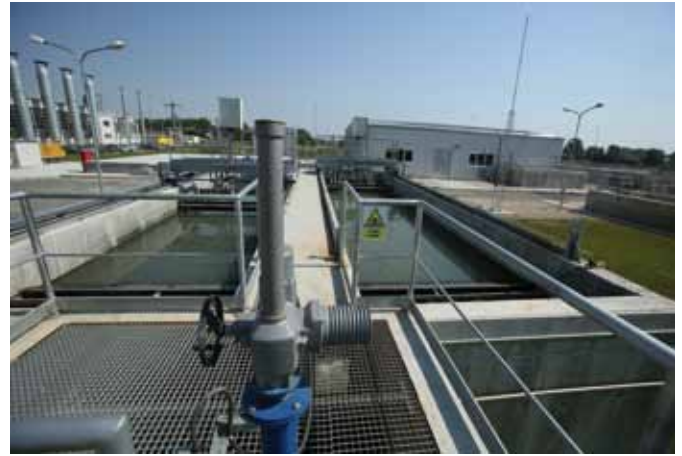
▲ TURNKEY PROJECTS OF THE WASTE WATER TREATMENT PLANTS IN ZIMNICEA, AGNITA AND DUMBRAVENI
