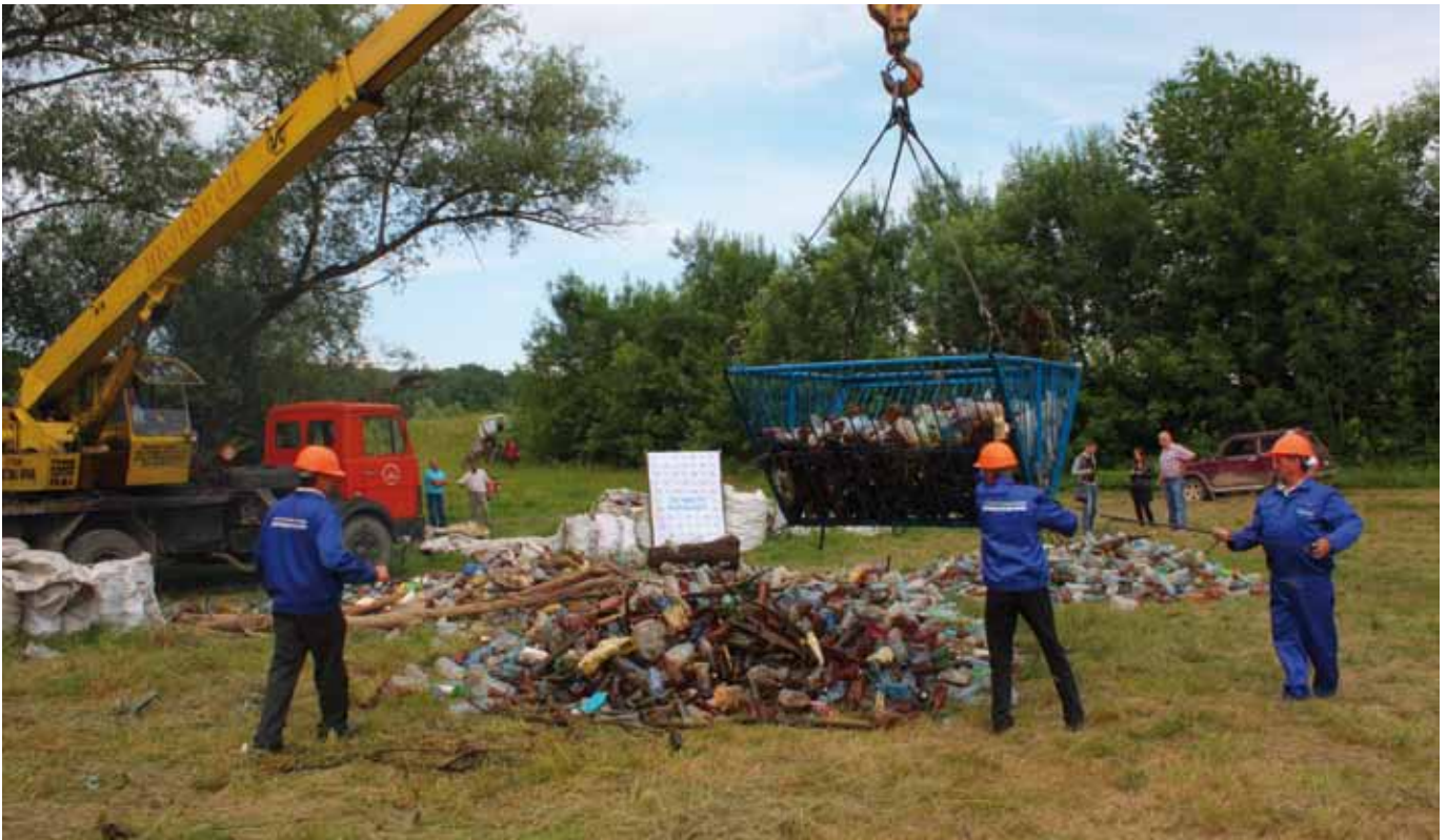
▲ DESIGN AND WORKS SUPERVISION FOR THE CONSTRUCTION OF MECHANICAL WASTE SEPARATION FACILITY IN THE CITY OF GRODNO IN BELARUS
