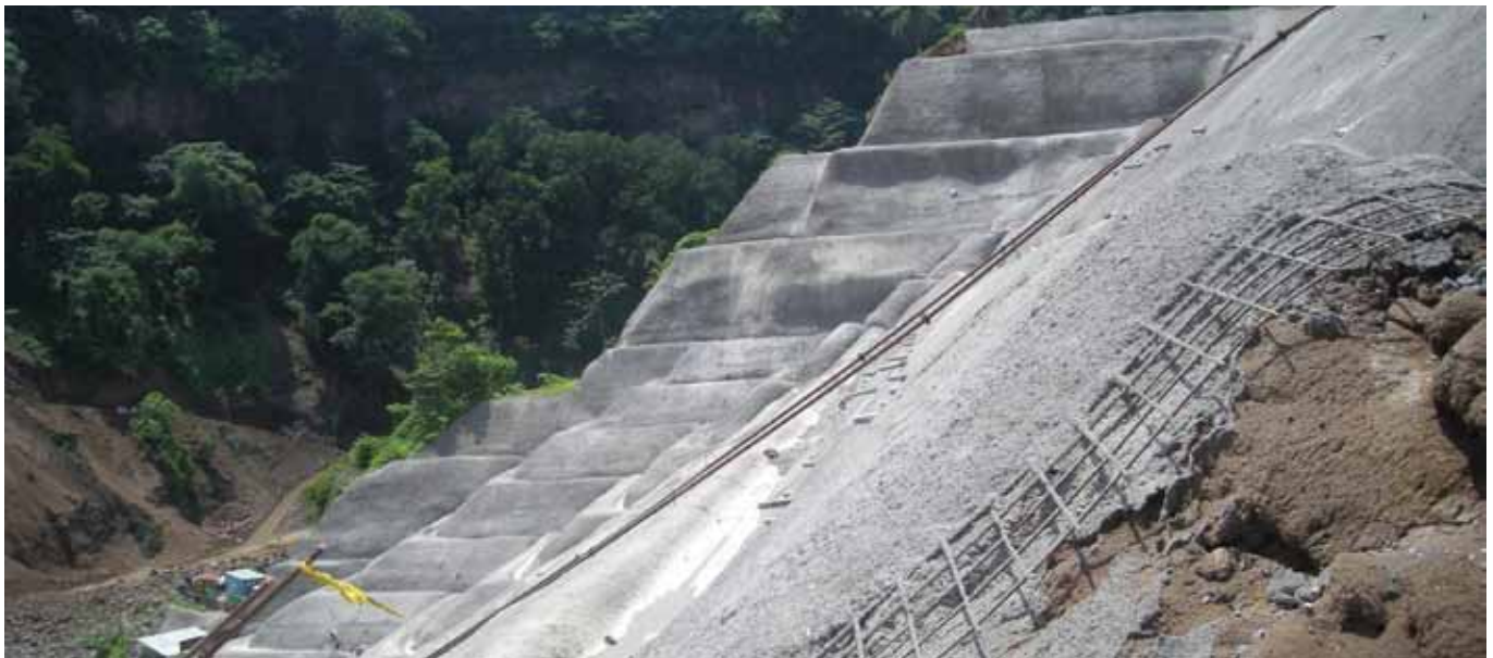
▲ AUSCULTATION AND GEOTECHNICAL CONTROL OF THE SLOPE LOCATED NEXT TO TARCOLES DAM IN COSTA RICA
