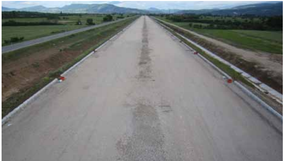
▲ SUPERVISION OF THE CONSTRUCTION WORKS ON THE HIGHWAY E-80 IN SERBIA
