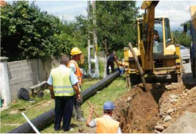
▲ EXTENSION AND MODERNISATION OF WATER AND SEWERAGE INFRASTRUCTURES IN GIURGIU, OLT AND GORJ COUNTIES
