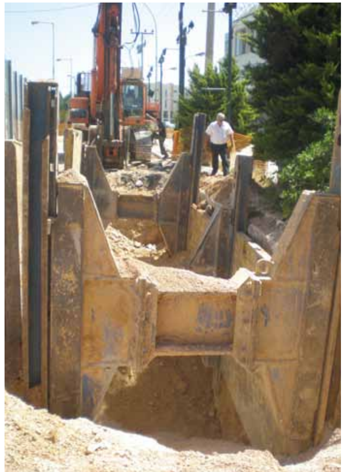
▲ SEWERAGE NETWORK, E.S.P.EL PROJECT
