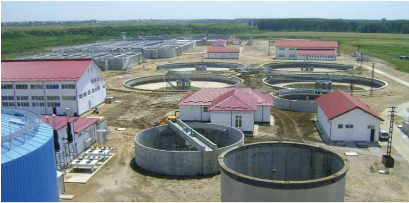
Rehabilitation and extension of the drinking water and wastewater infrastructure in Dolj County in Romania
