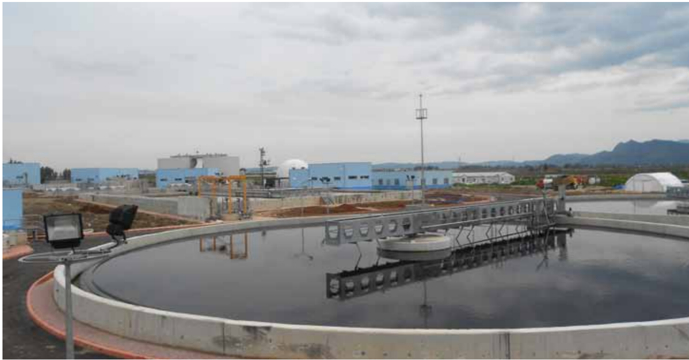
Supervision of construction works for the Ceyhan waste water and stormwater project in Turkey
