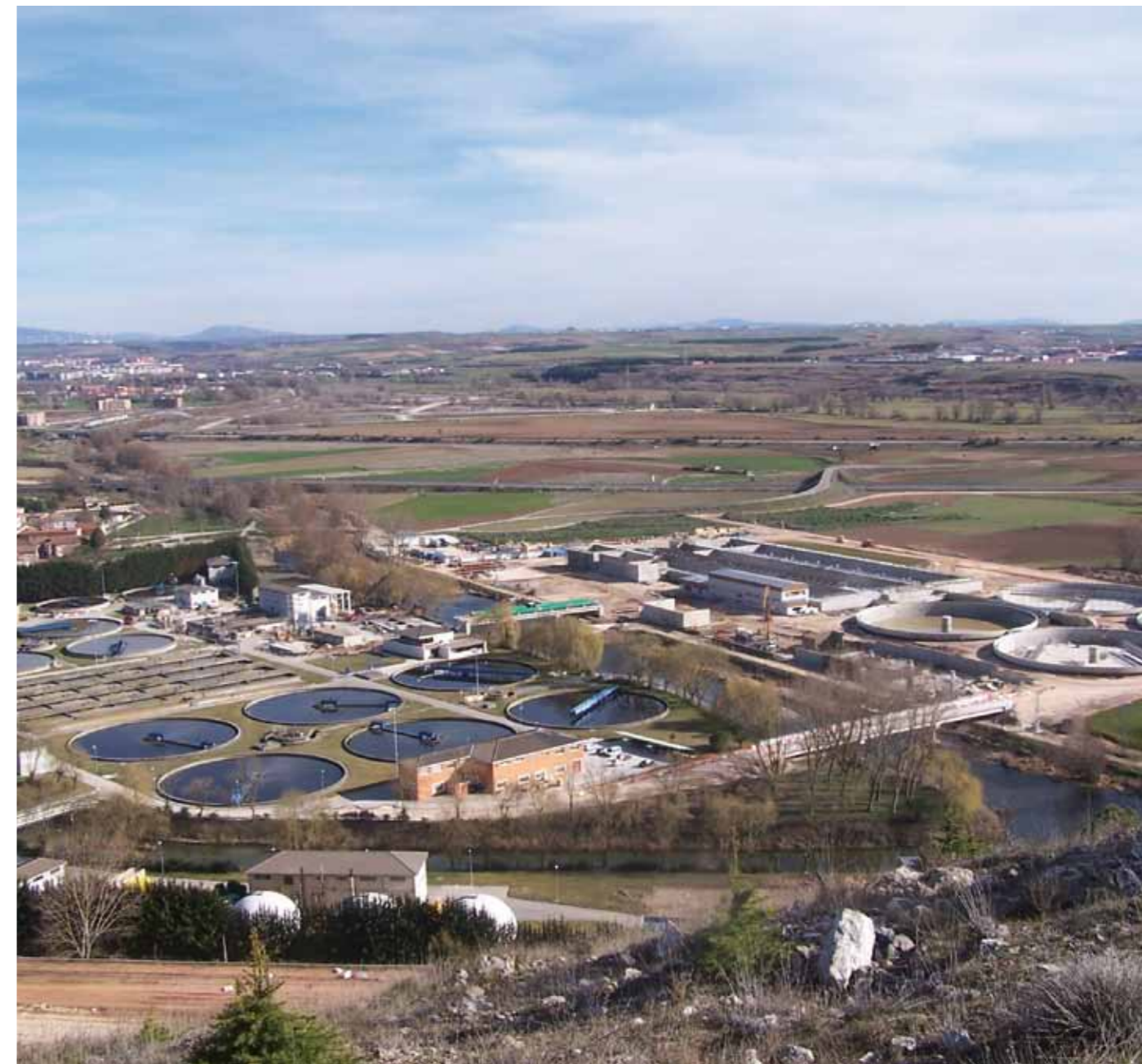
Enlargement of the Wastewater Treatment Plant of Burgos
