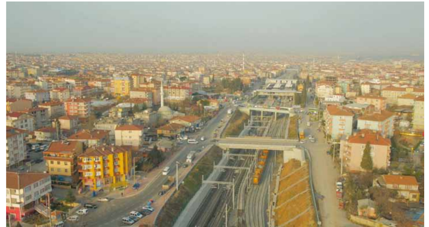
Marmaray Project: Gebze-Haydarpaşa Line, Sirkeci-Halkali In Istanbul, Turkey
