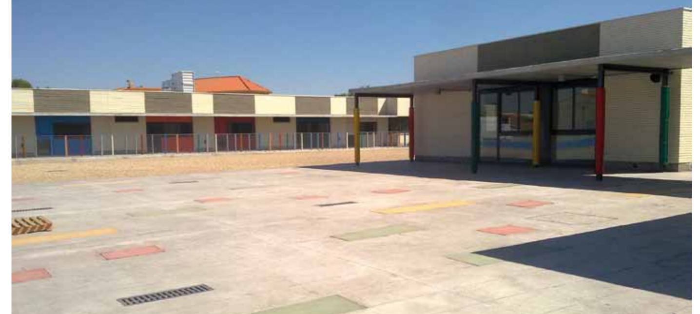
Quality control of the construction of a school in Toledo
