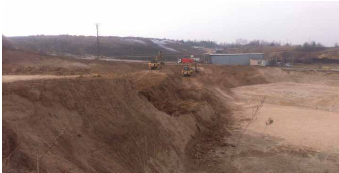
Integrated solid waste management system project, City of Grodno
