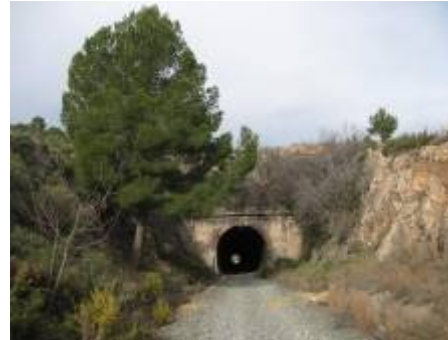
Santa Bárbara Tunnel
