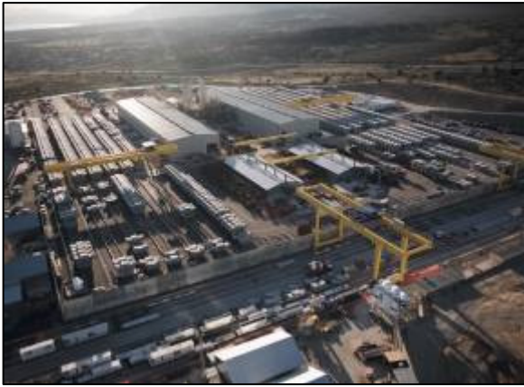
Ariel view of the ring segment manufacturing plants. Boca Sur.
